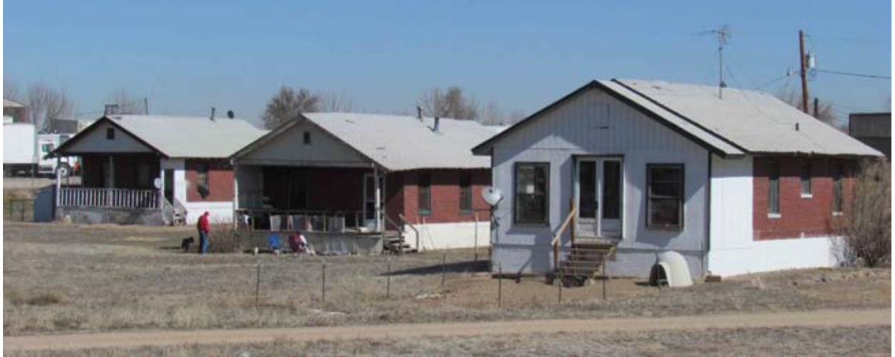
Work Camp Houses opposite Roller Rink
