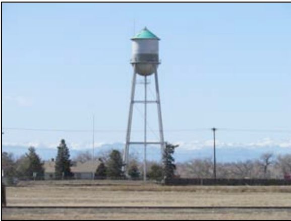
Kuner Water Tower
